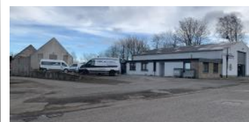
GRC Aquatech Improvements to the old depot site
