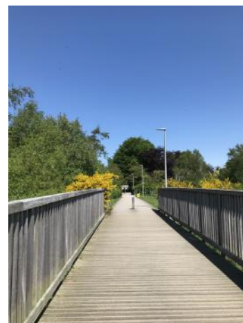
Bridge at the Health Centre and Hospital
